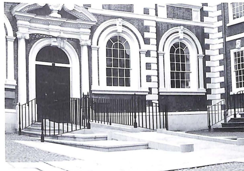
New Bluecoat Ramp
